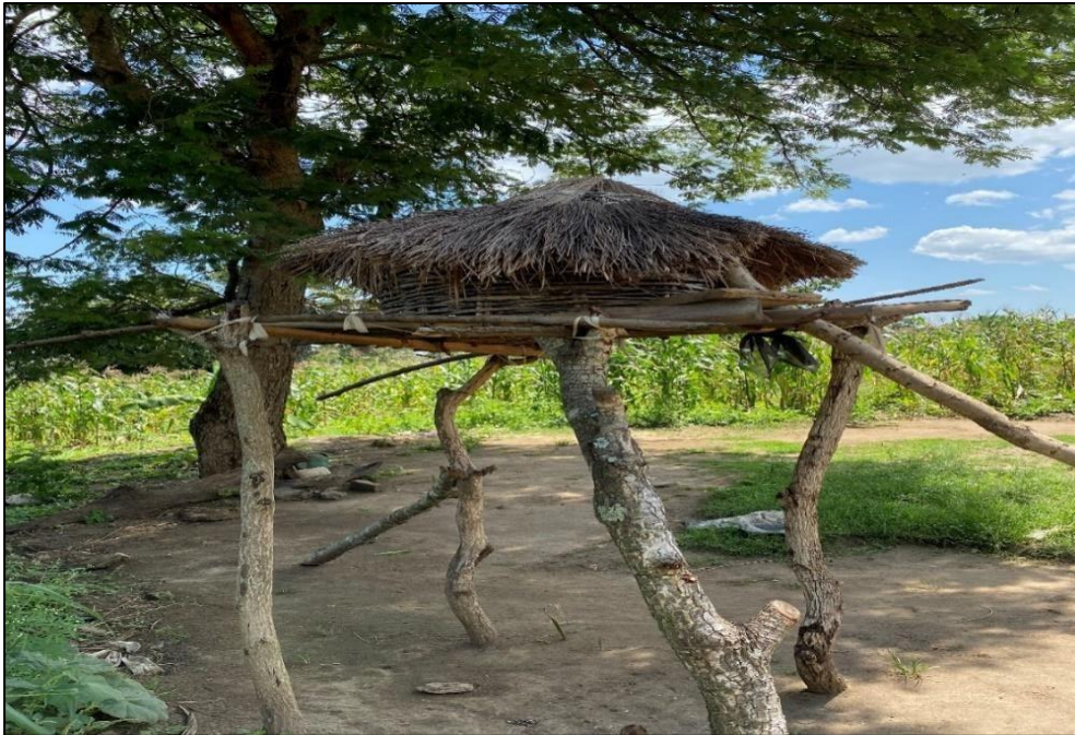
Figure 9. Shows a traditional food storage facility in one of the refugee homes.
