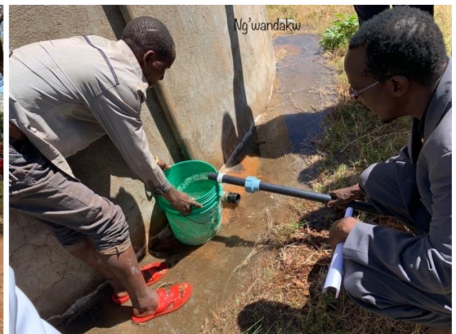
An Engineer from RUWASA's Mbulu district office measuring water flow entering into the Tank
