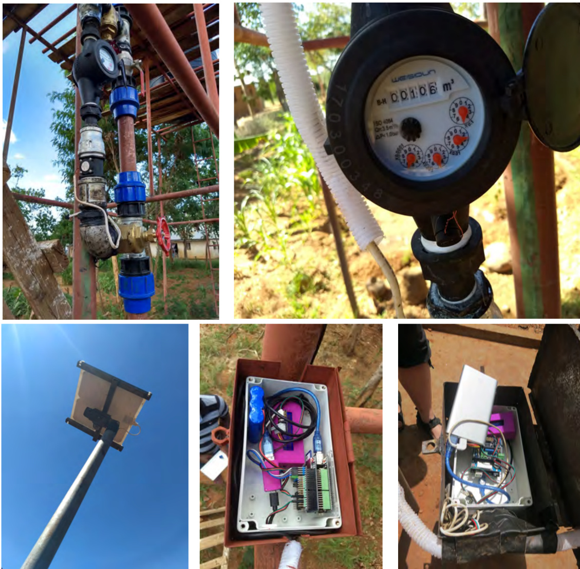
Figure 2.26: Remote monitoring system installed in 2018 by NCA as described by Martinsen [2018, p. 30-31]
