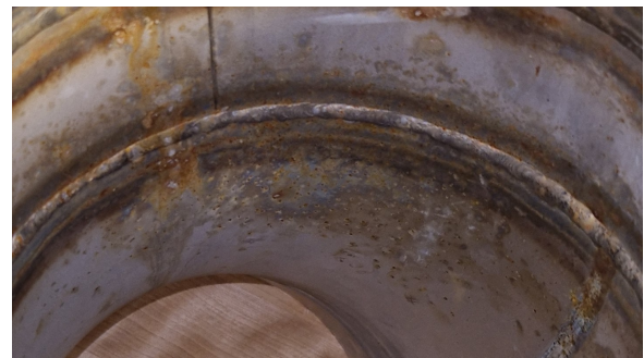
(b) Inside of pipe
