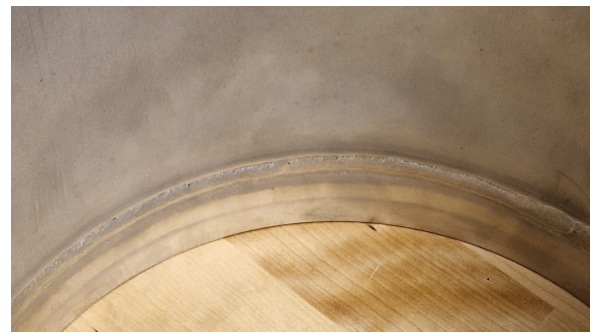
(b) Inside of pipe
