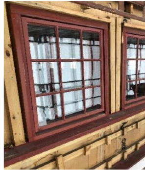
Figure 37 Intervention on the façade of Skur 38, with previous windows and the new installation. (Taken from FutureBuilt Skur 38 https://www.futurebuilt.no/Forbildeprosjekter?municipal%5B%5D=oslo# )
