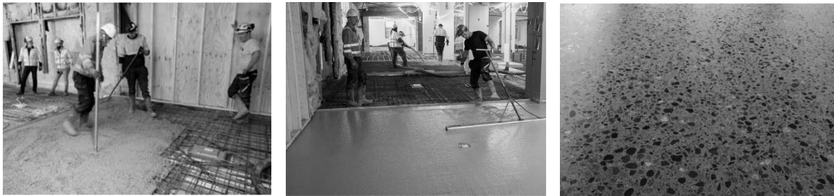
Figure 30 Visual documentation of Skur 38 intervention to the ground floor
