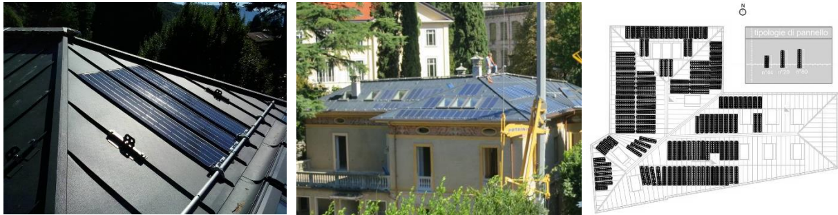
Figure 25 Solar panels implementation in Villa Castelli (Bellano), Italy. (Taken from Historic Building Energy Retrofit Atlas – HiBERAtlas )
