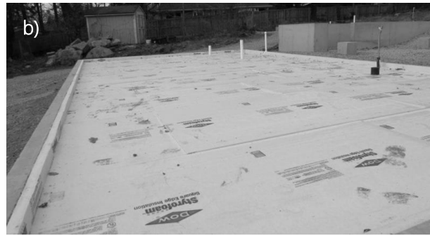
Figure 32 a) Technical detail of a usual upgrading of a concrete slab with insulation (Taken from Housing Retrofit: Ground floor insulation) b) Image of an insulation installation in a former garage to become a habitable space. (Taken from How to Insulate an Existing Concrete Slab https://todayshomeowner.com/insulation/guides/how-to-insulate-an-existing-concrete-slab/ )
