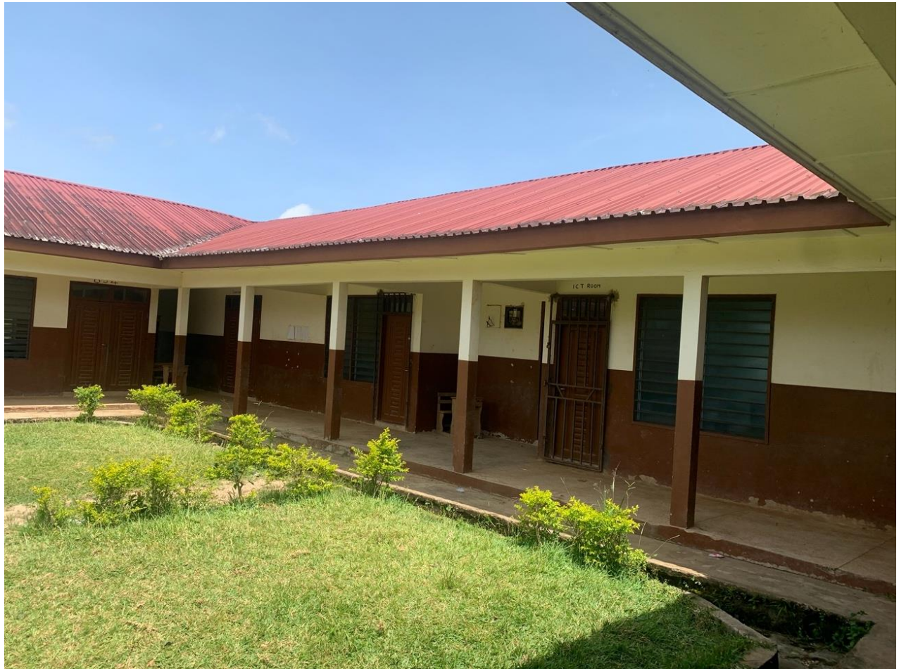
Figure 7. Public school building in Adelekezo
