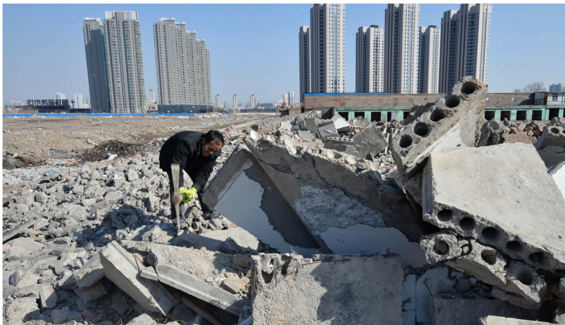
Figur 7: Betong knuses (Biørnstad, 2016).
