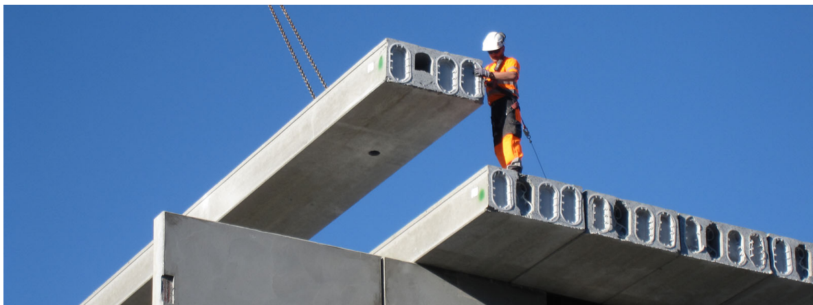
Figur 8: Hulldekke i betong (Loe Betongelementer AS, 2023).
