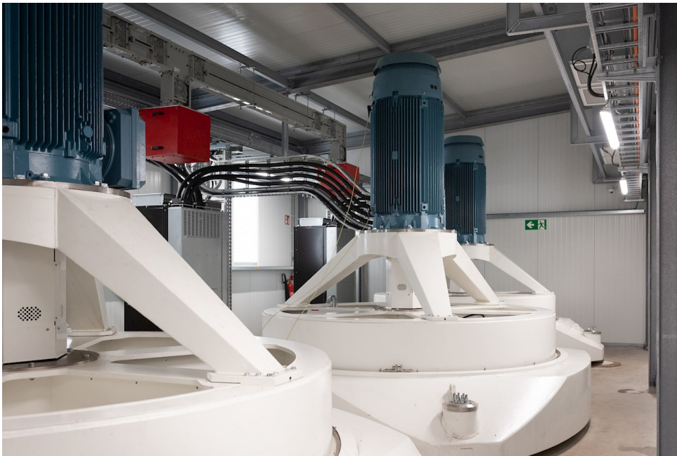
Figure 1.5: ABB and S4's flywheels that stabilizes the Dutch grid [2].
