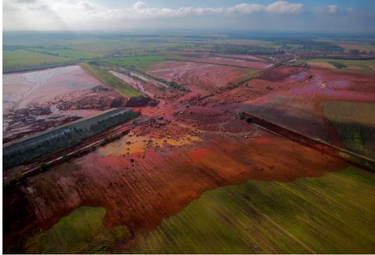
Figure 2: Aerial view of the broken dyke near Ajka, Hungary [14].
