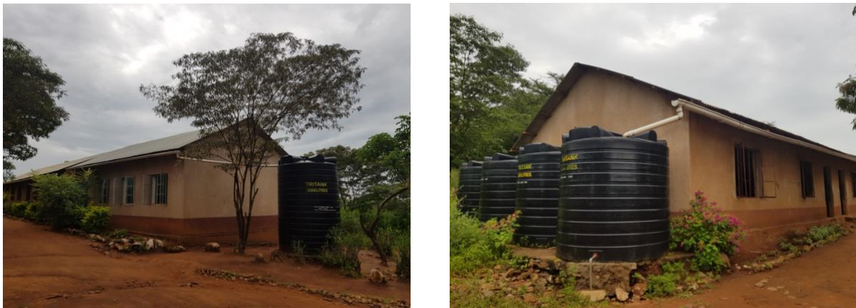
Figure 5.2: Rainwater harvesting system at Mewadani Primary school. Photos by: Vibeke Brandvold.
