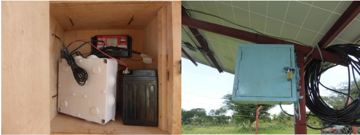
Figure 3.12: Inside of the wooden box (left). The wooden box was locked and installed under the solar panels in protection from sun and rain (right).
