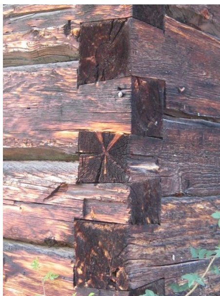
Figure 8: Dovetail joint exemplified in a building from Rendalen in Norway. Photo: Per Hvamstad/Anno Musea i Nord-Østerdalen.
