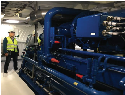
Figure 5 An ammonia system onboard a fishing vessel
