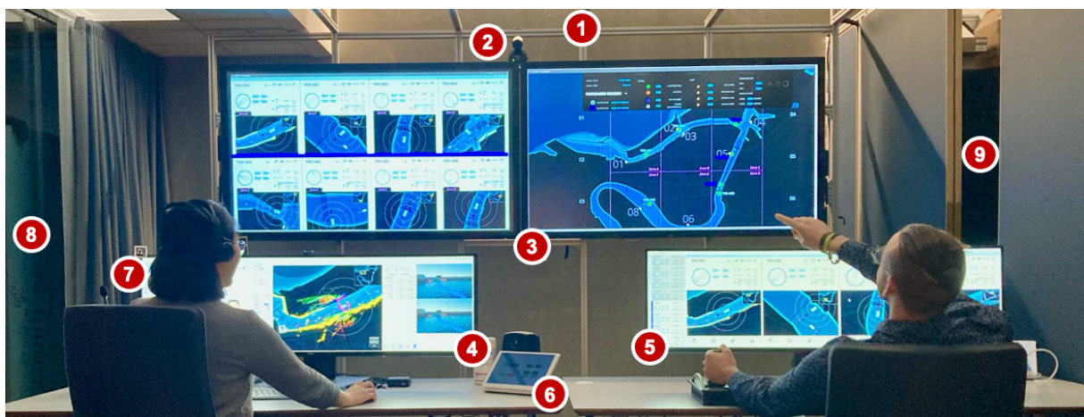
Figure 4: The control room with (1) Aluflex grid for flexibility, (2) cameras, (3) two height adjustable touch screens, (4-5) operator stations, (6) control panel, (7) microphones and loudspeakers, (8) view to observation room, (9) technical equipment (Photo: Erik Veitch)
