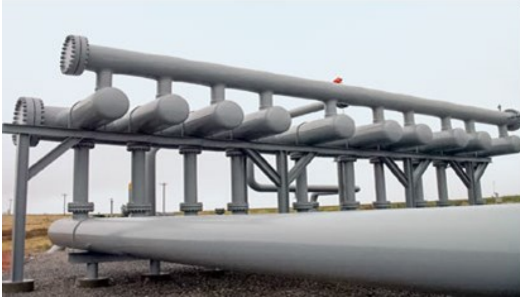
Figure 3-22: Parking loop type slug catcher taken from (Kalat Jari et al., 2015)
