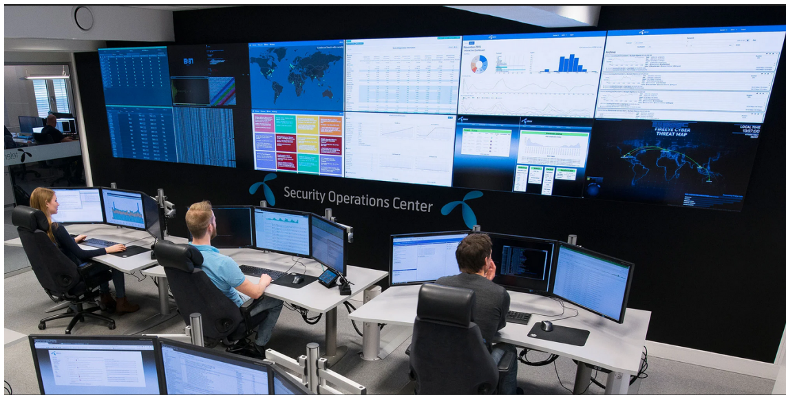
Figure 4: Security operation center at Telenor [4]
