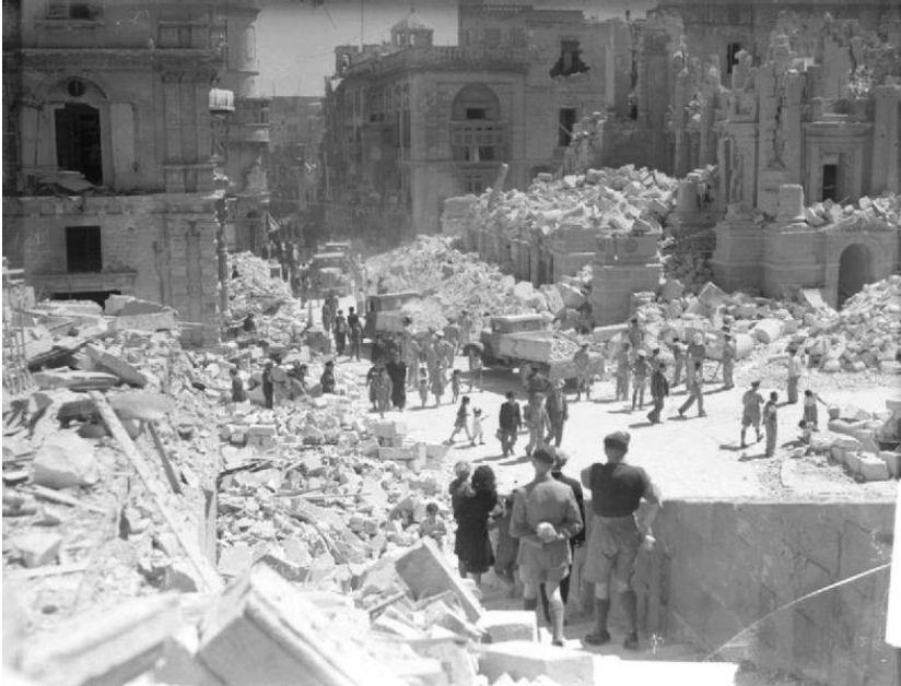
Figure 2-7 Bomb Damage in Valletta, Malta, 1 MAY 1942 (Source: https://www.iwm.org.uk )
