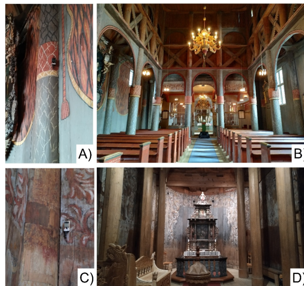
Figure A1. Indoor of Ringebu (B) and Heddal (D) stave churches: wooden building assets and altars are visible. The sensors positioned in Ringebu (A) and Heddal (C) are shown as well.
