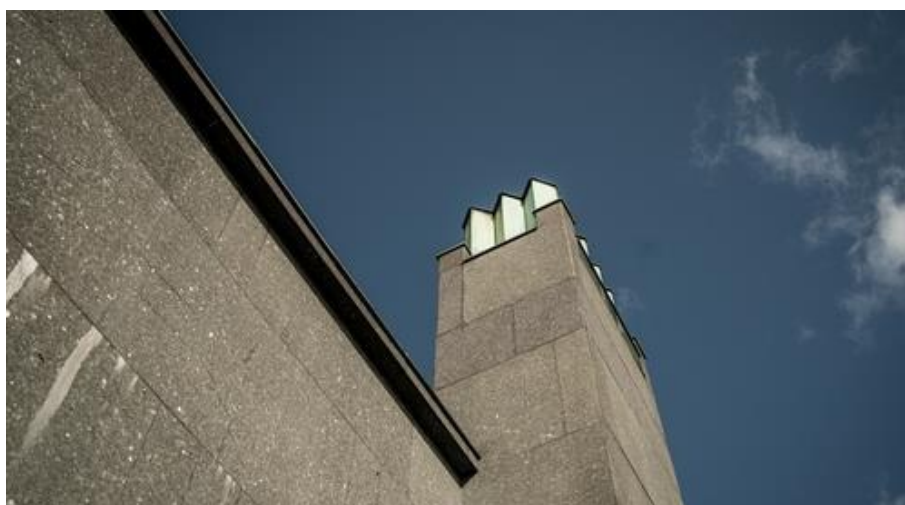
Figure 4.25: The natural quartzite stone façade cladding in KA23 ( https://www.ka23.no )
