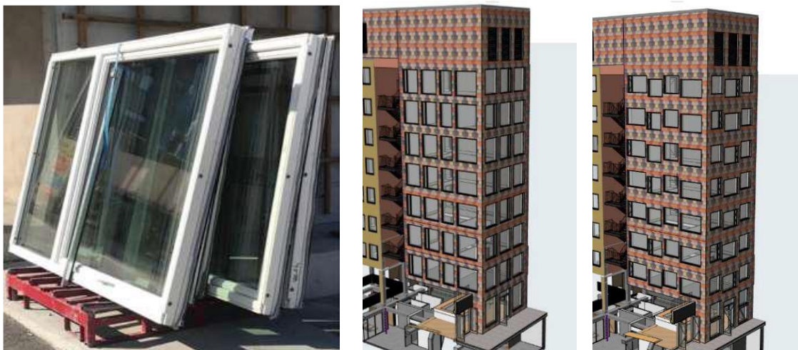
Figure 4.18: Windows dismantled from a housing project in Kværnerbyen Photo: Resirqel, Facade extension, designed with 1) New windows, 2) Used windows. Illustrations: MAD architects (Nordby et al., 2019)
