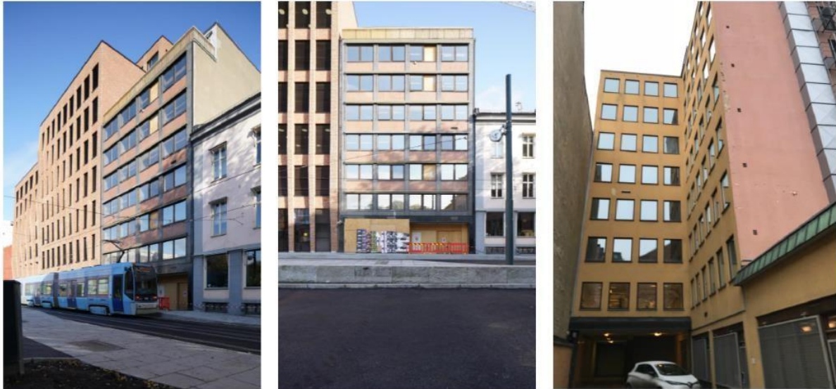
Figure 3.2: Kristian August gate 13 - existing building (Elverum, 2020)
