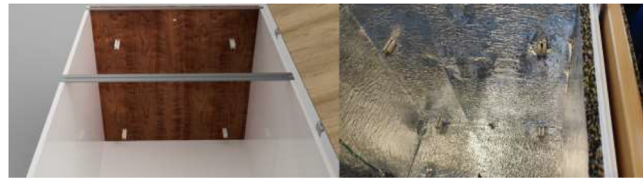
Fig. 18. Aluminum profile mounting.
