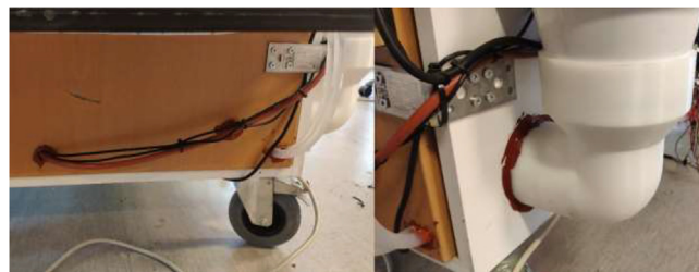
Fig. 21. HTS sealing of chamber heated cables (left) and exhaust fan (right).
