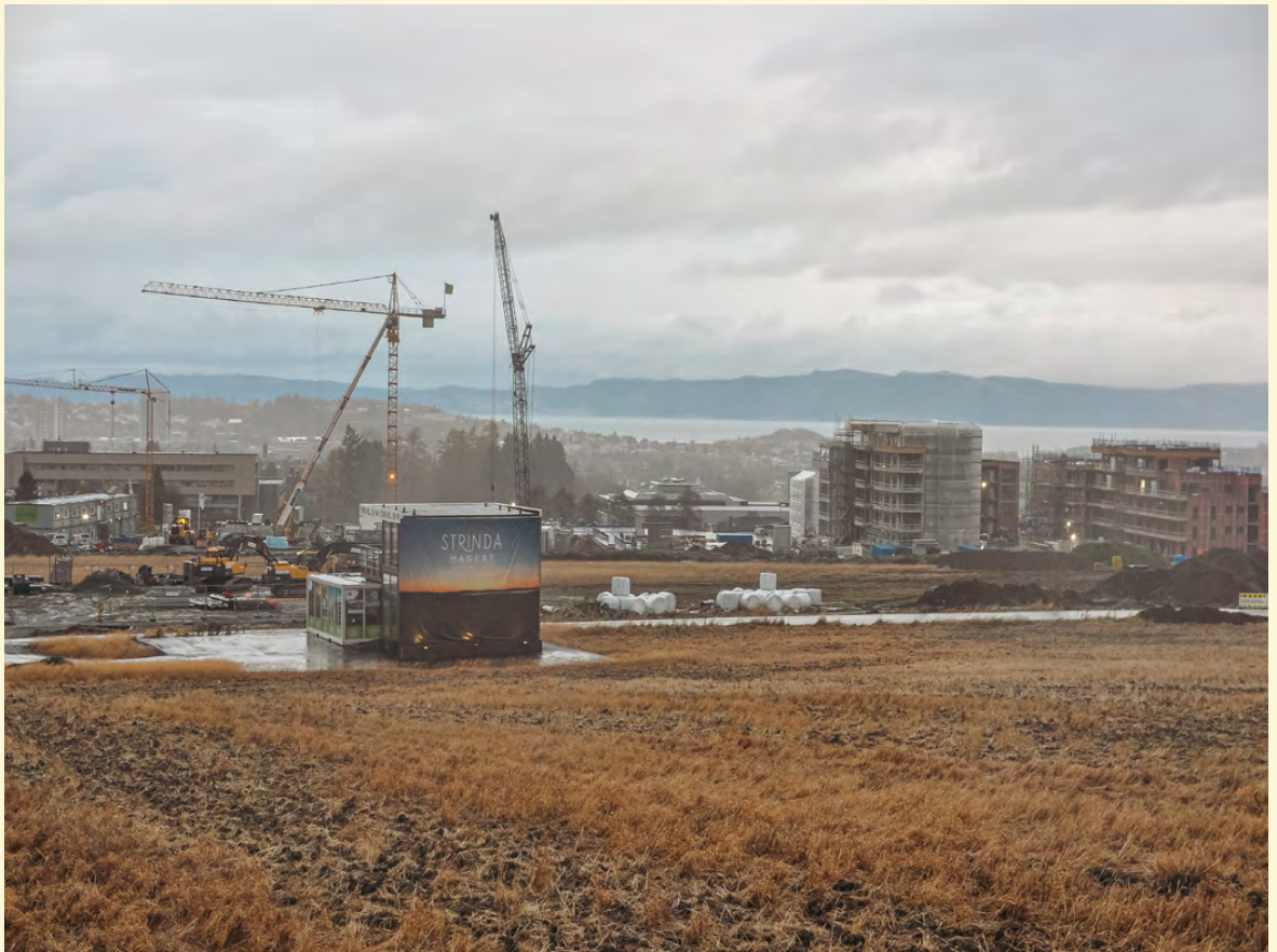
Garden city being constructed. Strinda Hageby
