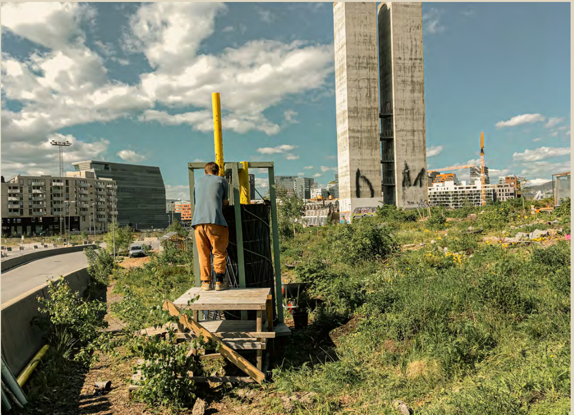
Removing the pipes for the second time
