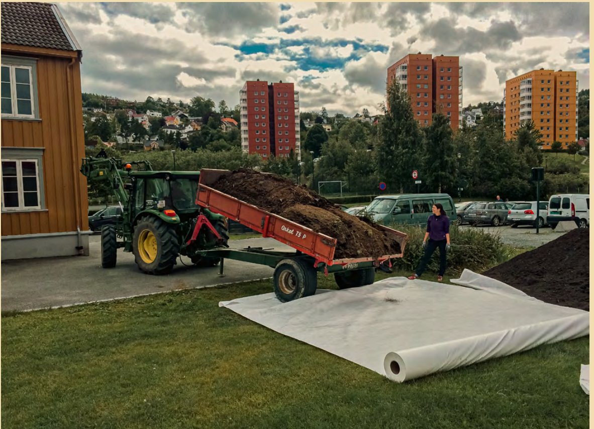
Unloading composted manure for the new mix
