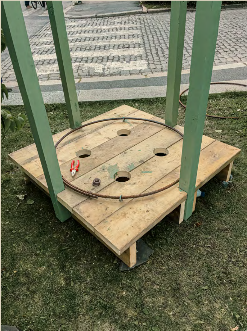
Drilling holes for the pipes
