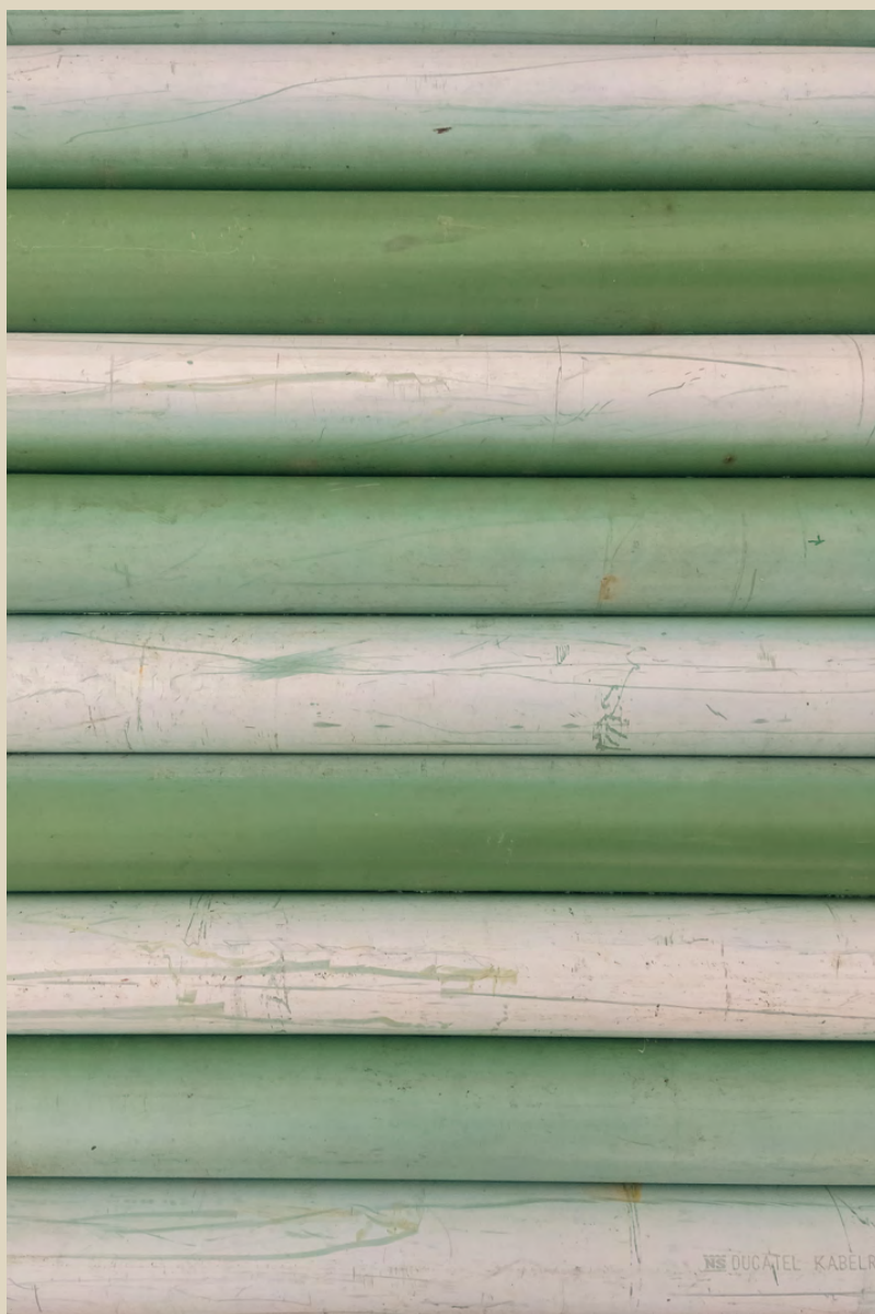
After filling the reactor we cut the pipes in two to make a roof.
