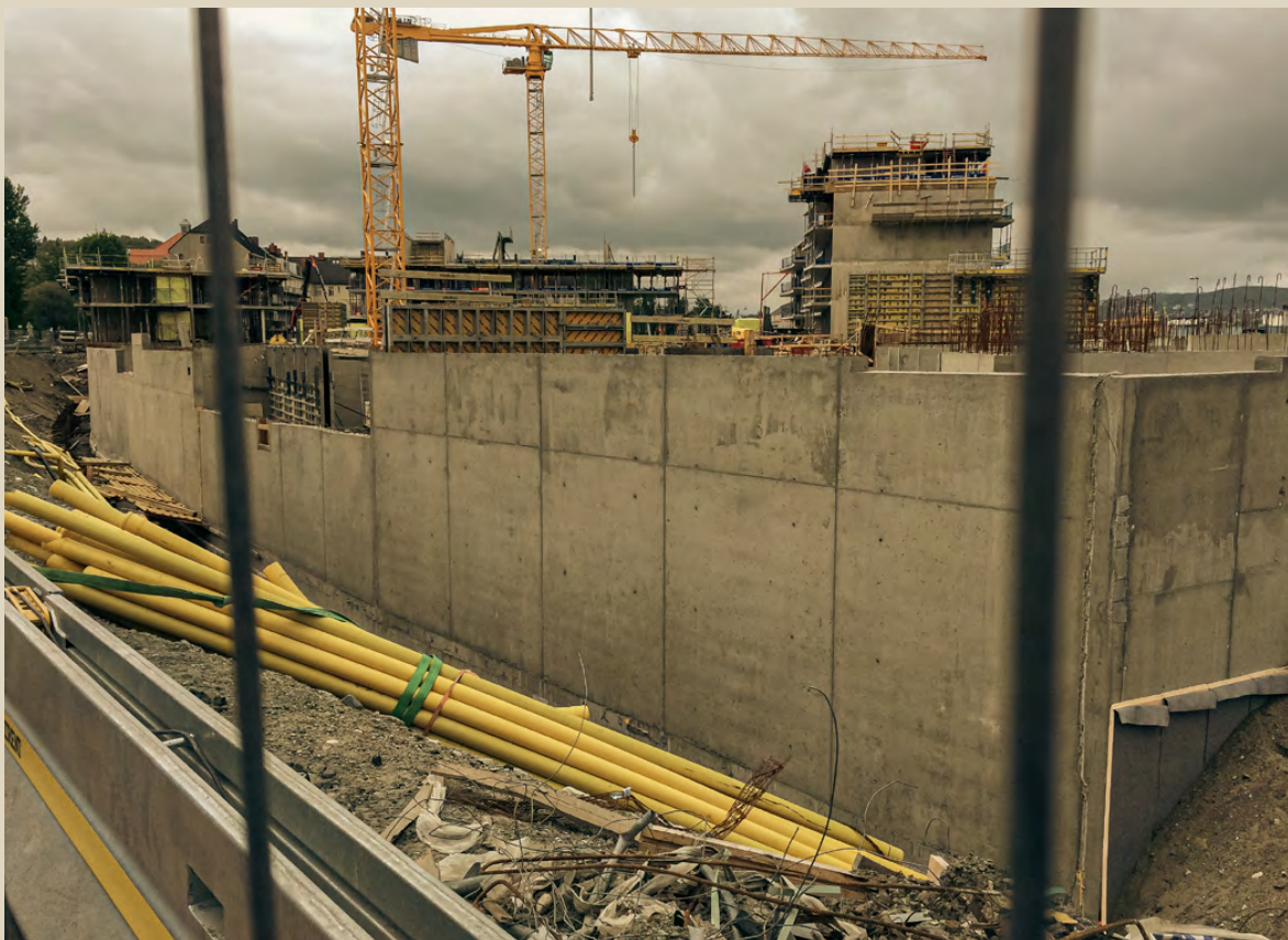
Biking around in the city looking for pipes with 120mm diameter.
