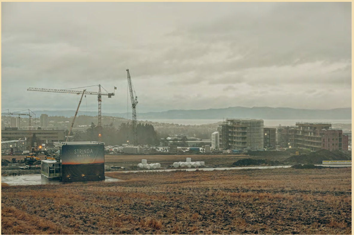
Strinda hageby (Garden City) being constructed
