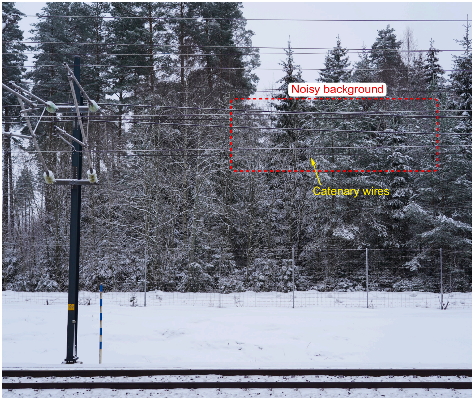
Fig. 5. Wire detection challenge caused by noisy background.
