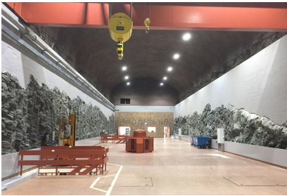
(a) Generator hall in Bratsberg hydropower plant.
