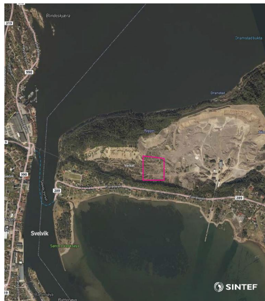
Figure 2.1: Aerial view of the sand and gravel ridge (the Svelvik ridge) where the Field Laboratory is located (Eliasson, 2020)
