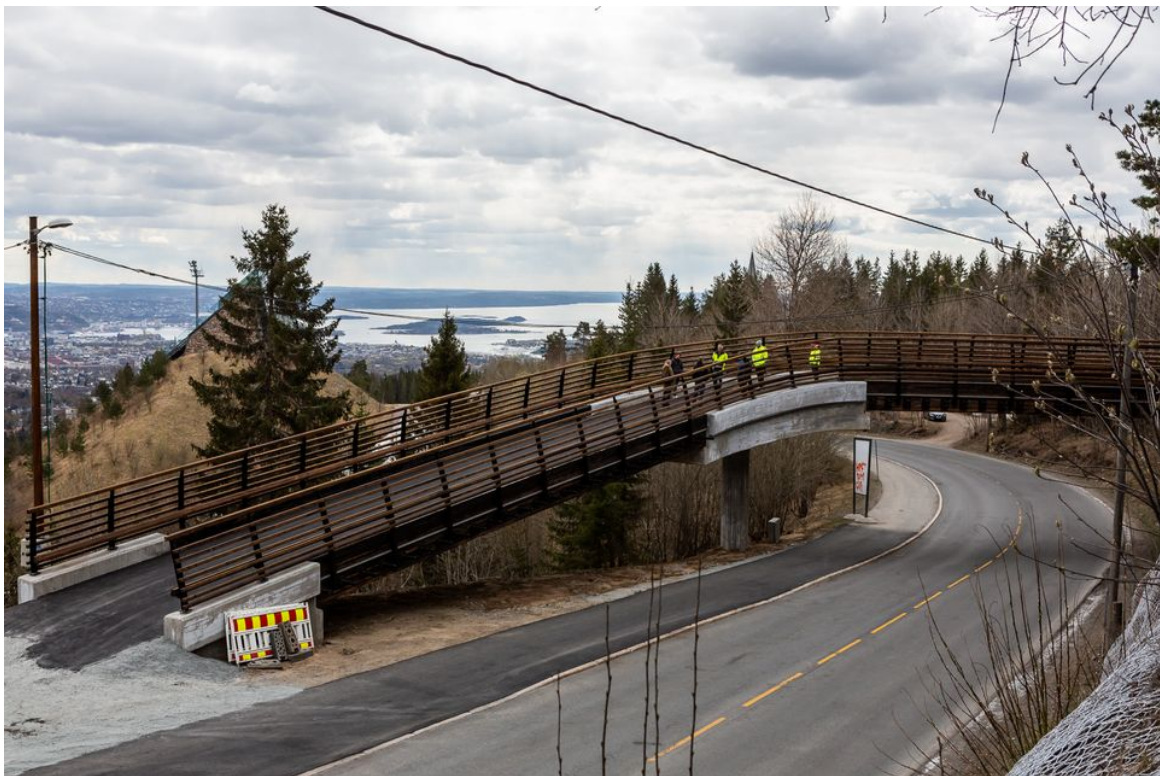
Figure 2.1: Example of a SLT bridge in Holmenkollen [17].
