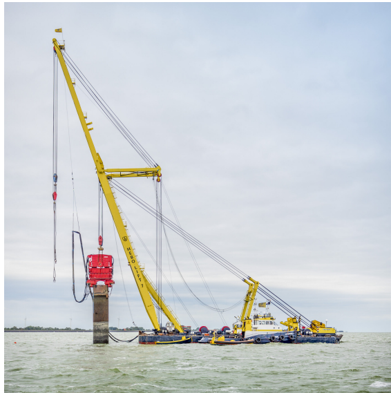
Figure 2.4: Decommissioning Lely Offshore Wind Farm
