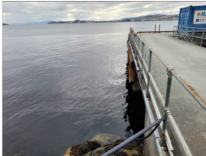
Figure 29: Sample 1 location: Pier at TBS.
