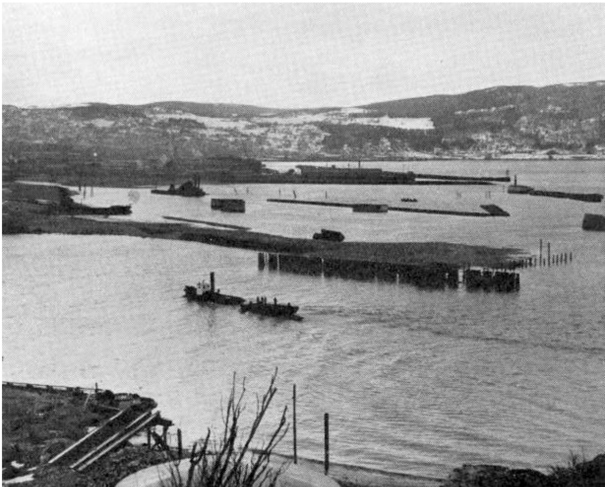
Figure 14: Pier II under development in 1949 (Trondheim Havn, 2022)
