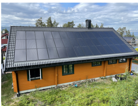
Figure 2.1: The solar panel installation in Asker
