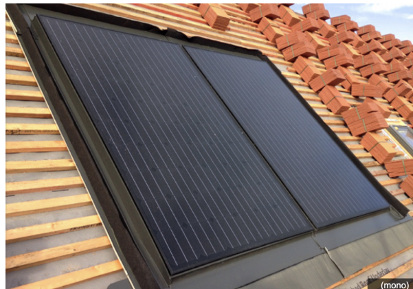
Figure 3.1: Viridian Fusion PV16-300 300Wp Mono panel[8]
