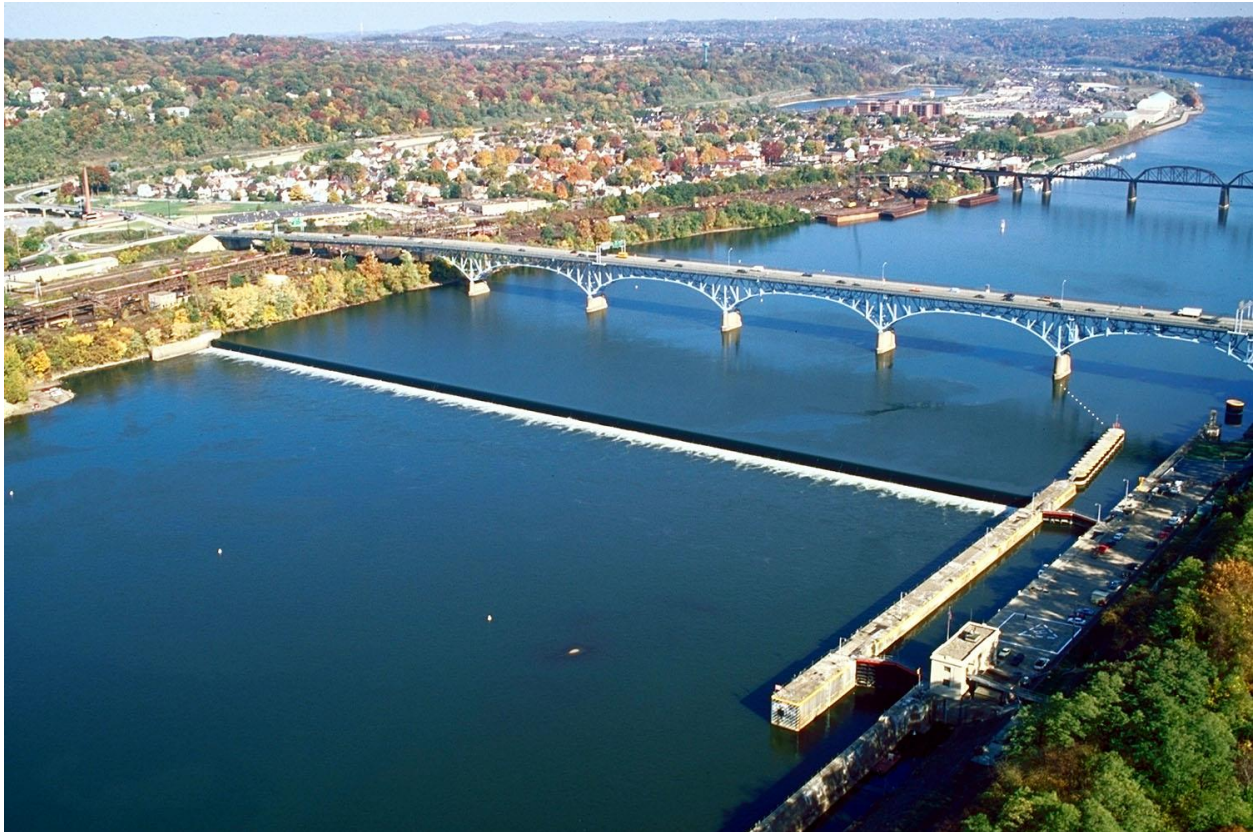
Figure 10: USACE lock and dam 2 Allegheny river next to Sharpsburg borough ( USACE,1993)
