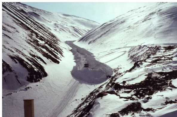
Figure 8.2: Picture of how the snowpack in Vannledningsdalen is prepared to minimise the slush flow risk using trenching. The same picture is presented in Section 6.4, but repeated here to improve readability. Source: Jónsson and Gauer [92].
