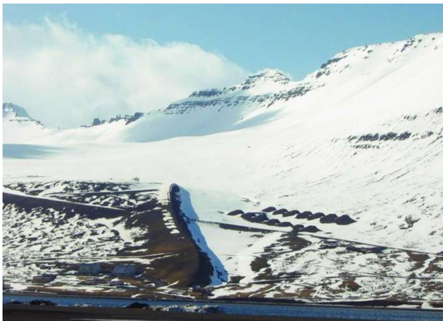
Figure 6.6: Deflecting dam and retarding cones at Seljalandsmúli in Ísafjörður, northwestern Iceland. Source: [59, p. 117]. Photo: Tómas Jóhannesson.
