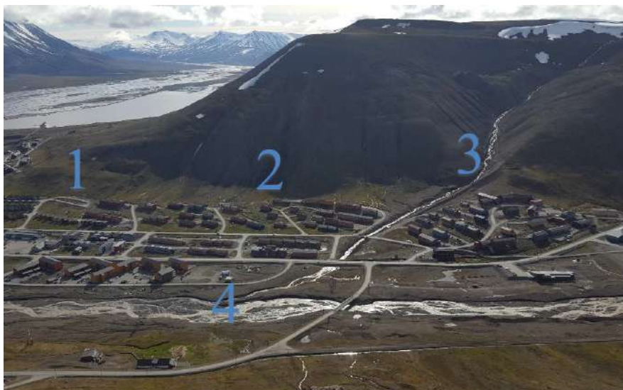
Figure 7.1: Photo giving an overview of Longyearbyen centre including the areas of interest for mitigation measures. 1 - Lia above Spisshusene (residential houses) where snowdrift fences, support structures and a catching dam have been constructed. 2 - Sukkertoppen and Lia residential area where a catching dam and support structures are planned as mitigation measures against snow avalanches. 3 - Vannledningsdalen where flexible net barriers are planned as a mitigation measure against slush flows. 4 - Longyearelva where measures have been completed to avoid erosion and flooding. Source: Hoseth et al. [5].
