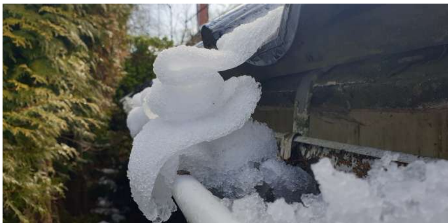
Figure 2.10: Viscous movement of spring snow gliding down a roof and folding in the roof gutter. Cohesive properties are also shown by the fold hanging over the edge. Photo: Haldis Døvlø Kalland.
