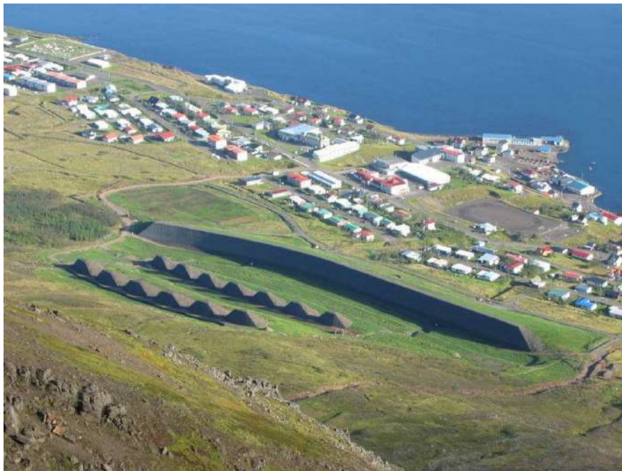
Figure 6.7: Photo of braking mounds in Neskaupstaður, Iceland, and the catching dam behind them. Each mound is 10 m high and the catching dam is 17 m high. Source: [90].
