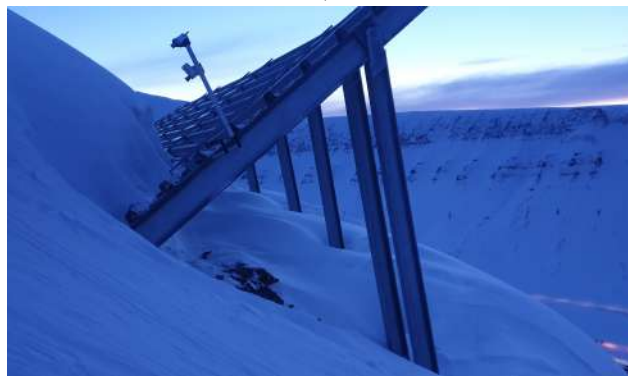
Figure 7.14: Support structures on Sukkertoppen photographed during field work on March 6 th 2022 showing how the snow cover is affected by wind transport of snow. a) A wind slab between the two upper lines of support structures photographed from below, b) Most the snow has been blown away between the supporting surface and supports. Photos: Haldis Døvre Kalland.
