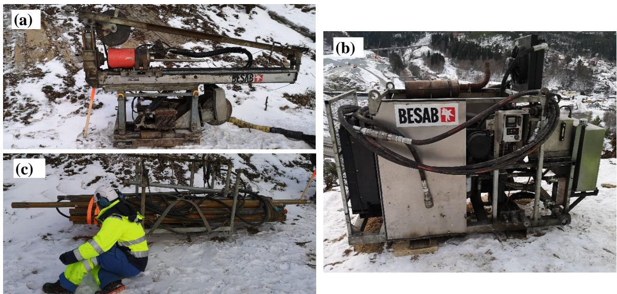
Figure F.2: Equipment used for drilling by Besab AB.
