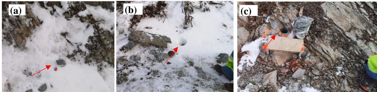
Figure F.1: Surface conditions at boreholes 1A, 4A, and 5A (from left to right). Drilling of boreholes 5X was not started at the time of inspection.
