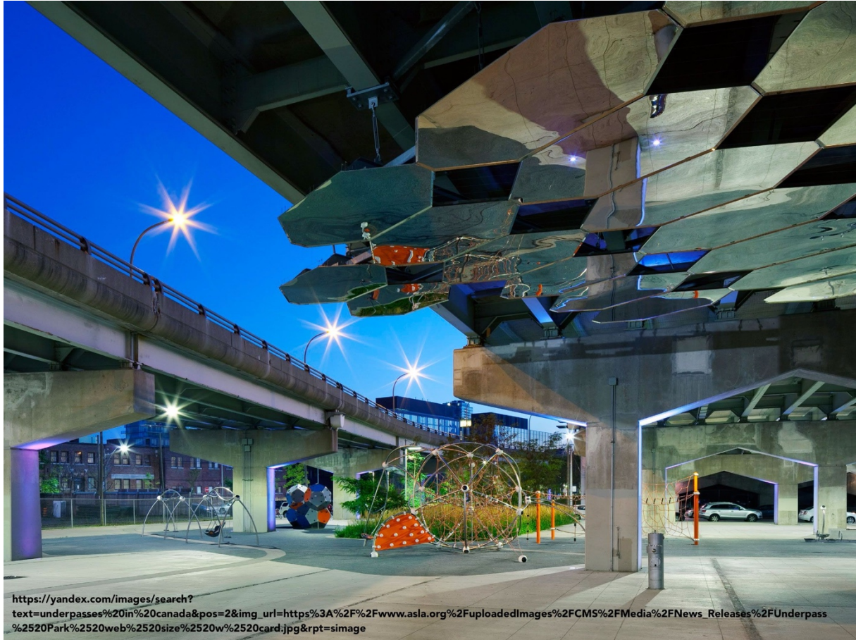
Figure 6.13: Underpasses in Canada
