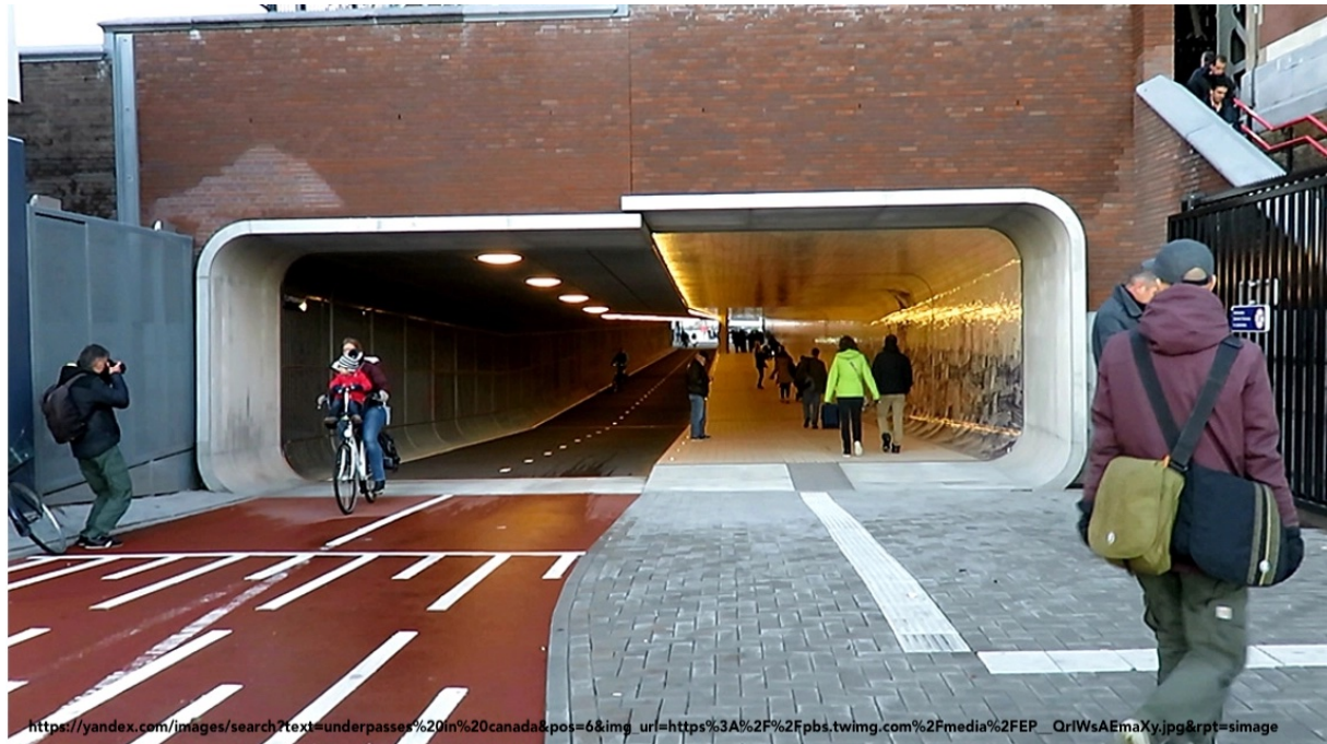
Figure 6.14: Underpasses in Netherlands
