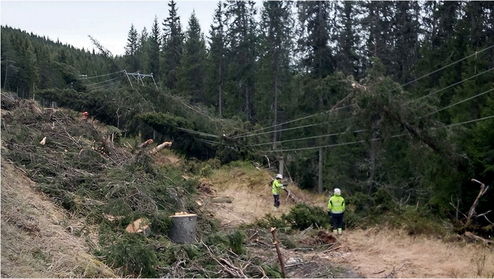
Figure 2.5: Photo of trees causing a power failure during the extreme weather in Vestfold and Telemark. Photo provided by an informant.
