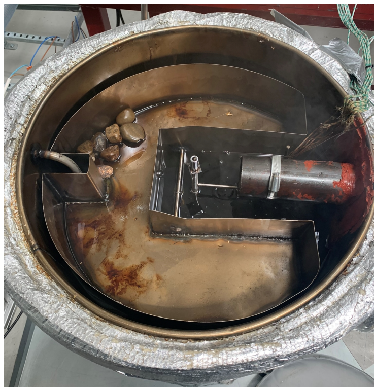
Figure 5.6: Displacement valve and top of pump in modified SHTES
