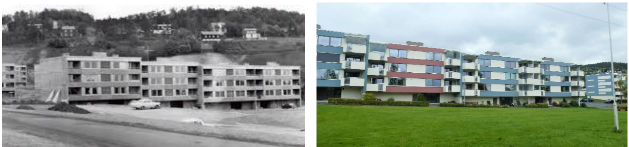
Figure 2.3 Othilienborg BL photographs; before extension of the balconies (left), after the extension of balconies (right).
