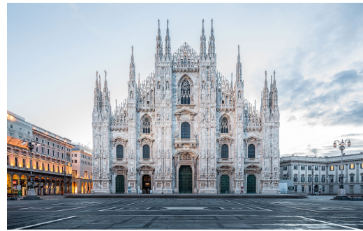
(b) As Duomo di Milano shows, Gothic cathedrals introduced spires and pointed arches. Image by Simone Simone.
