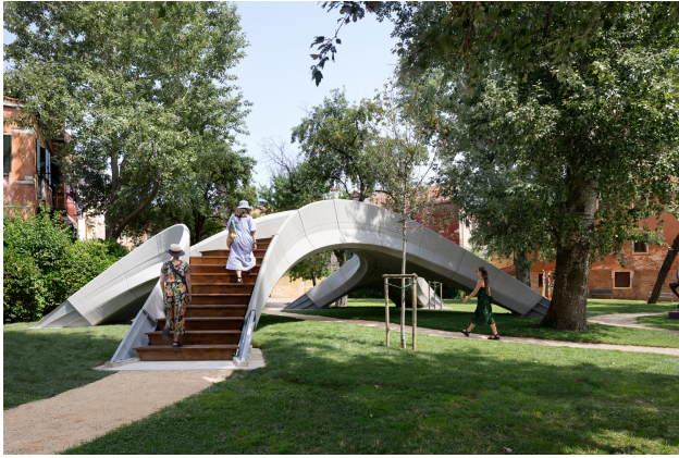
Figure 2.9: Striatus bridge assembled and in use. Image by naaro
