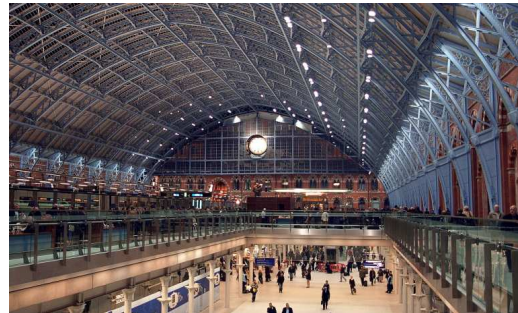
(d) Implementation of iron enable long spans for the St. Pancras station in London. Source: ('10 Things to Do at London's St Pancras', n.d.)
