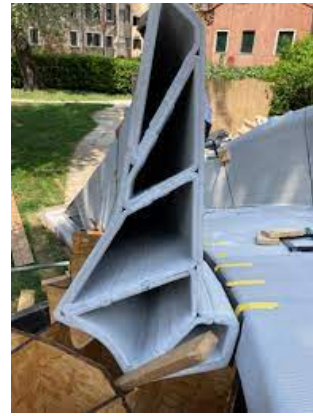
Figure 2.10: The hollow wedge shows the reduction of concrete. Image by Alessandro Dell'Endice.
