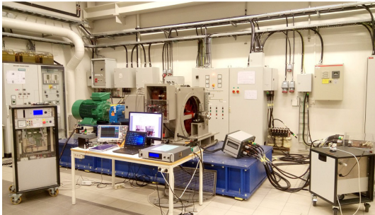
Fig. 8. Experimental test rig of a 100-kVA synchronous generator with 14 salient poles.
