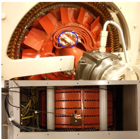
Fig. 2. Location of the shorted turns tap on the rotor (top) and the location of the stray magnetic field sensor installed on the stator backside of an SPSG.
