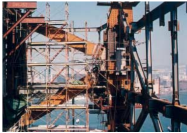
Figure 17: Bracing Hong Kong financial tower [32]
