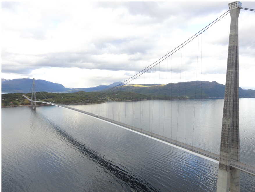
Figure 3.1: Picture of the Hålogaland Bridge. Courtesy of NTNU.
