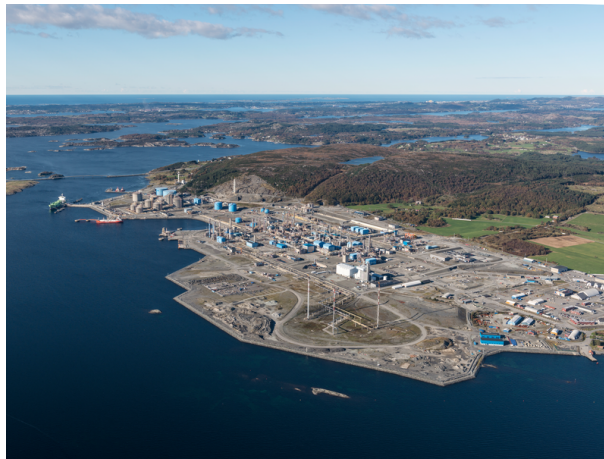
Figure 2.1.1: An overview of the Kårstø gas processing refinery in Rogaland, Norway. Picture taken by Markus Johansson / © Equinor.
