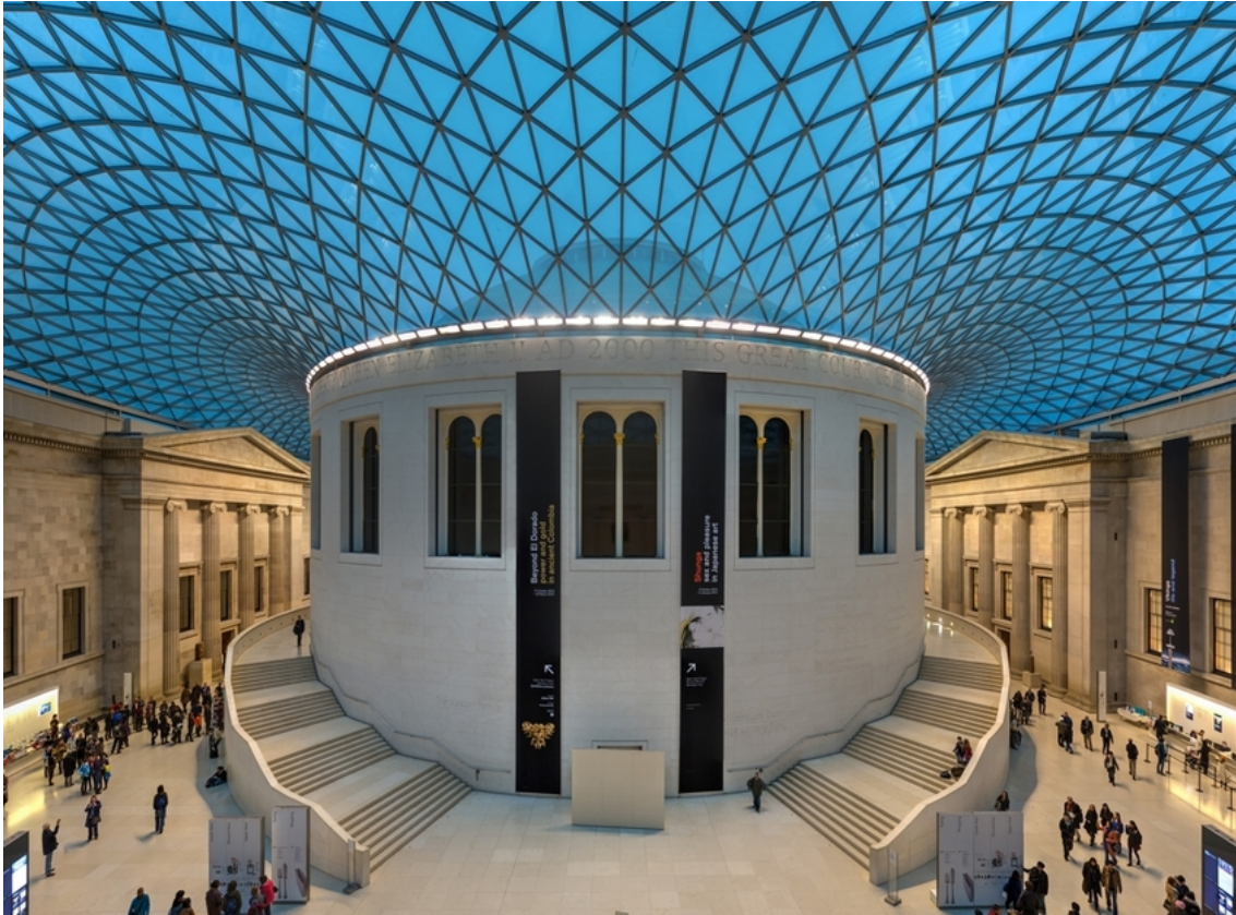
Figure 6.9: The gridshell roof over the Great Court in the British Museum (D'Amico, 2015).
