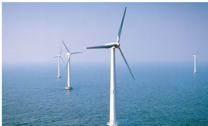
Figure 1.1: Vindeby wind farm in Denmark.
