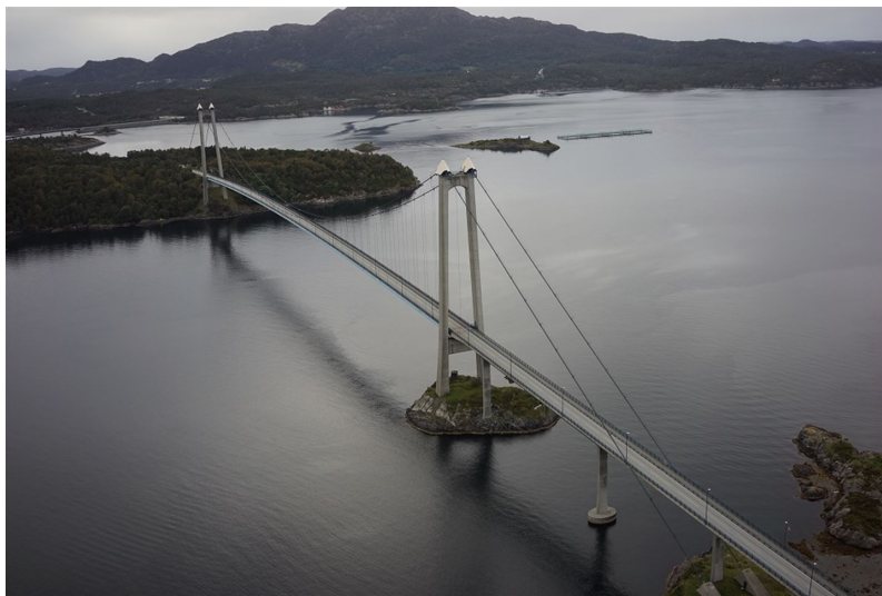
Figure 1: Bømla bridge in Vestland county in Norway. The bridge is in need of extensive and expensive maintenance (Ramstad 2022).
