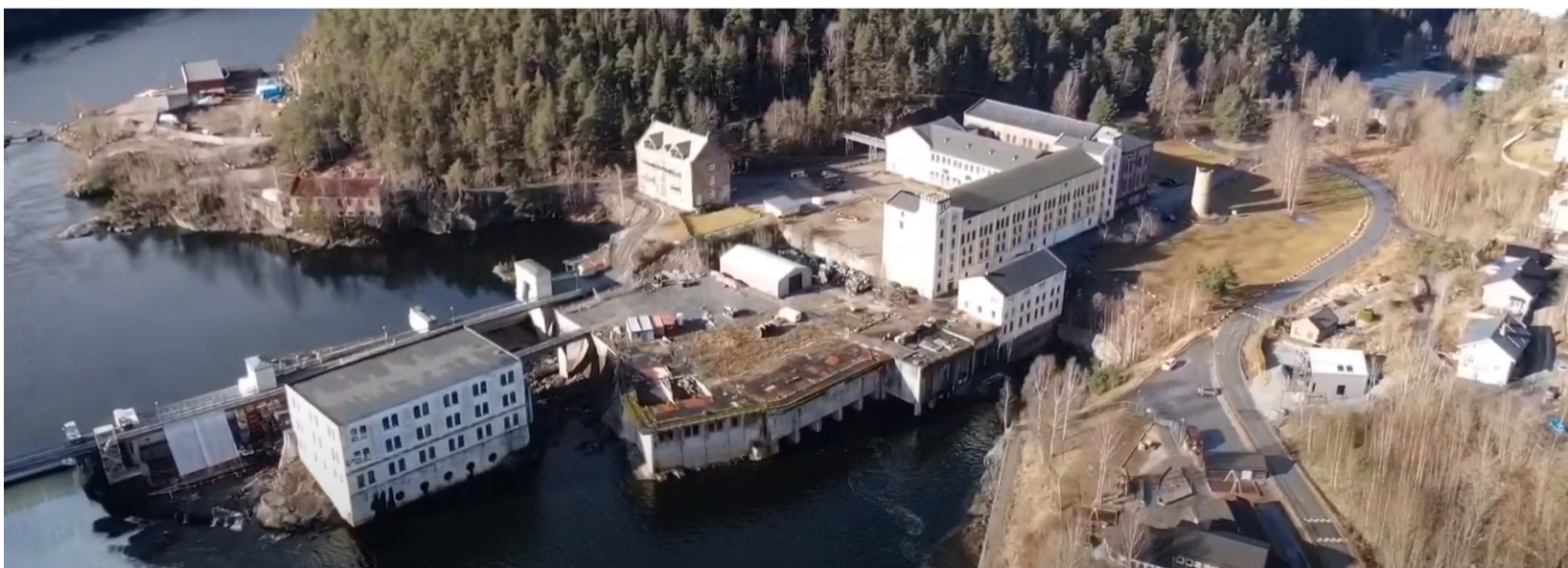
Figure 2 Present condition of Skotfossbruk
