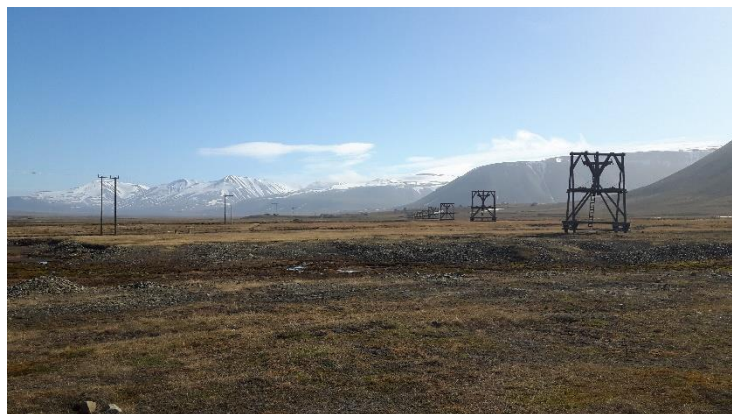
Figure 2: Part of the cableway in the Adventdalen valley. On the right: Wooden poles with artificial nest boxes.
