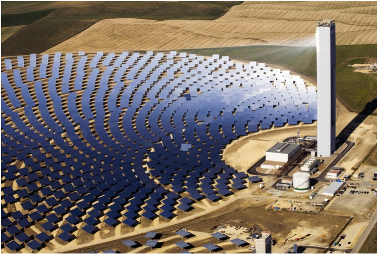
(a) Mirrors reflecting the light to a solar power tower in a CSP-plant [126]. (b) The tube collectors for hot water in a SHC-system [111].
