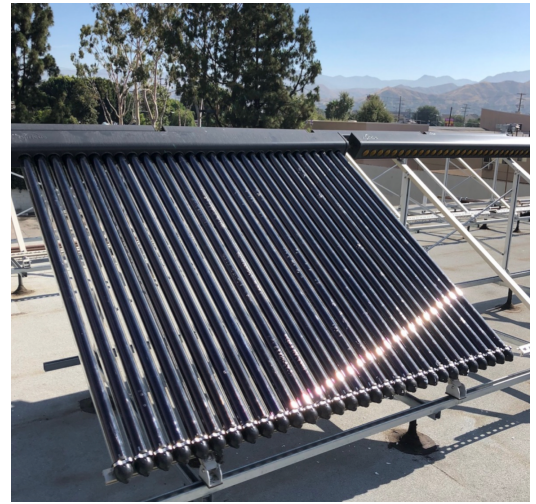
(a) Mirrors reflecting the light to a solar power tower in a CSP-plant [126]. (b) The tube collectors for hot water in a SHC-system [111].
