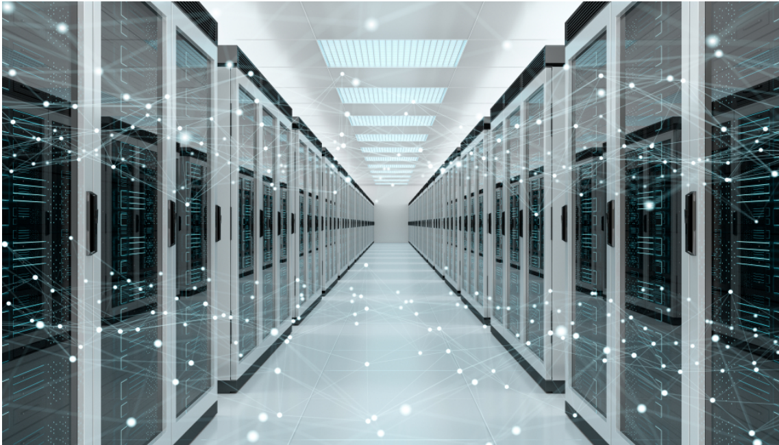
Figure 11: Inside a data center [46]
