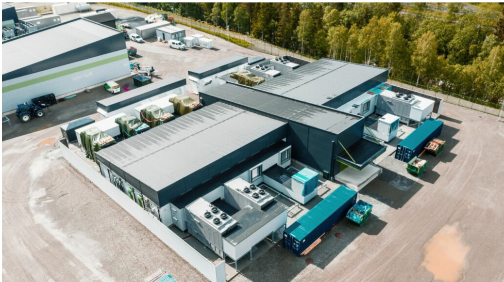
Figure 5: Volkswagen's data center in Rjukan [15]
