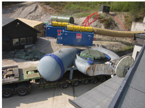
Figur 5: Trommel 110MVA generator, [4]
