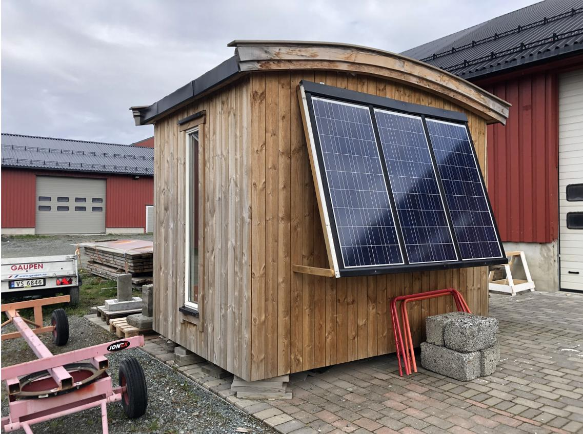
Figure 22: Solar panels in the opened position
