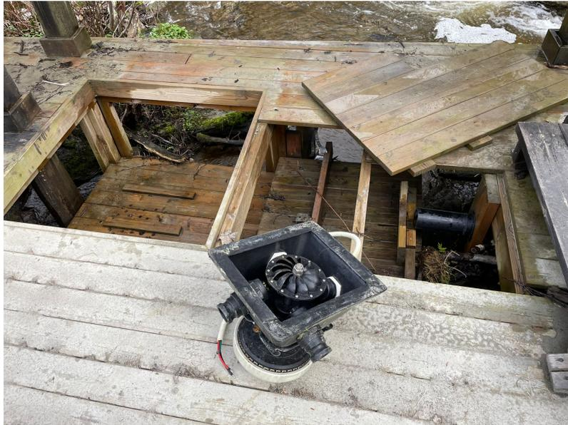
Figure 65: Hydro Turbine Generator Placement
