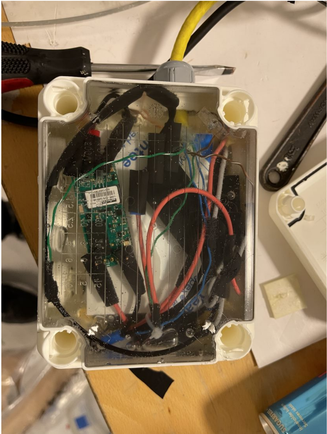
Figure 5.6: External box filled with epoxy.
