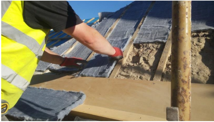
Figure 4.5: Installation of 20 mm aerogel blankets during rehabilitation (OldBuilders, n.d.)
