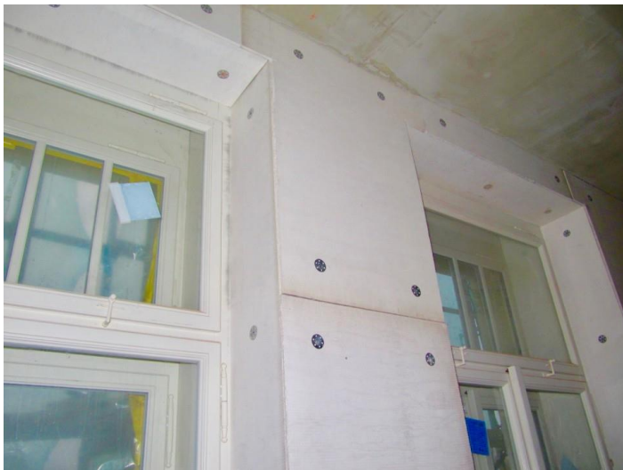
Figure 4.6: Aerogel thermaslim reveal board from Thermablok \lambda = 0.015 \text{ W}/(\text{mK}) (Thermablok, 2017d).
